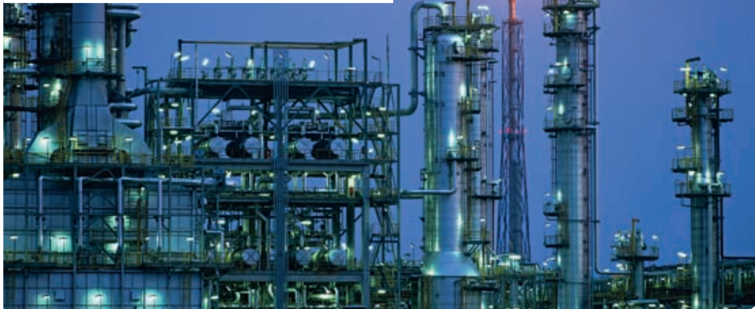
The new Chemical and Biotechnological Process Center CBP is being built in Leuna. © MEV
